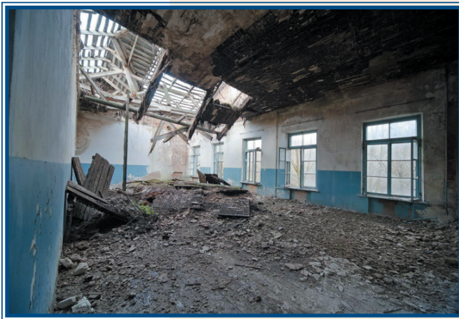
An abandoned building near the disaster sight. (Source: Semion Shevtsov)
