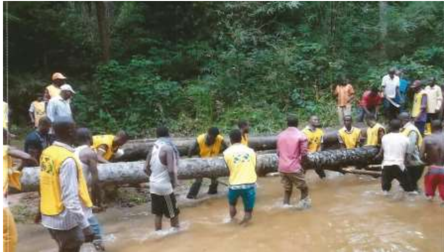
Figure 2: An example of Community Service: A Construction of bridge along Ikot Okwot-Oduo-Atang road, Nsit Ubium, Akwa Ibom State, Nigeria.
