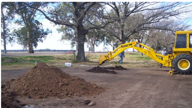
Picture 9. Soil removal tasks to monitor soil contaminated with hydrocarbons in a rural area and then remedied by stabilization methodologies (Alejo Ledesma, Argentina).
