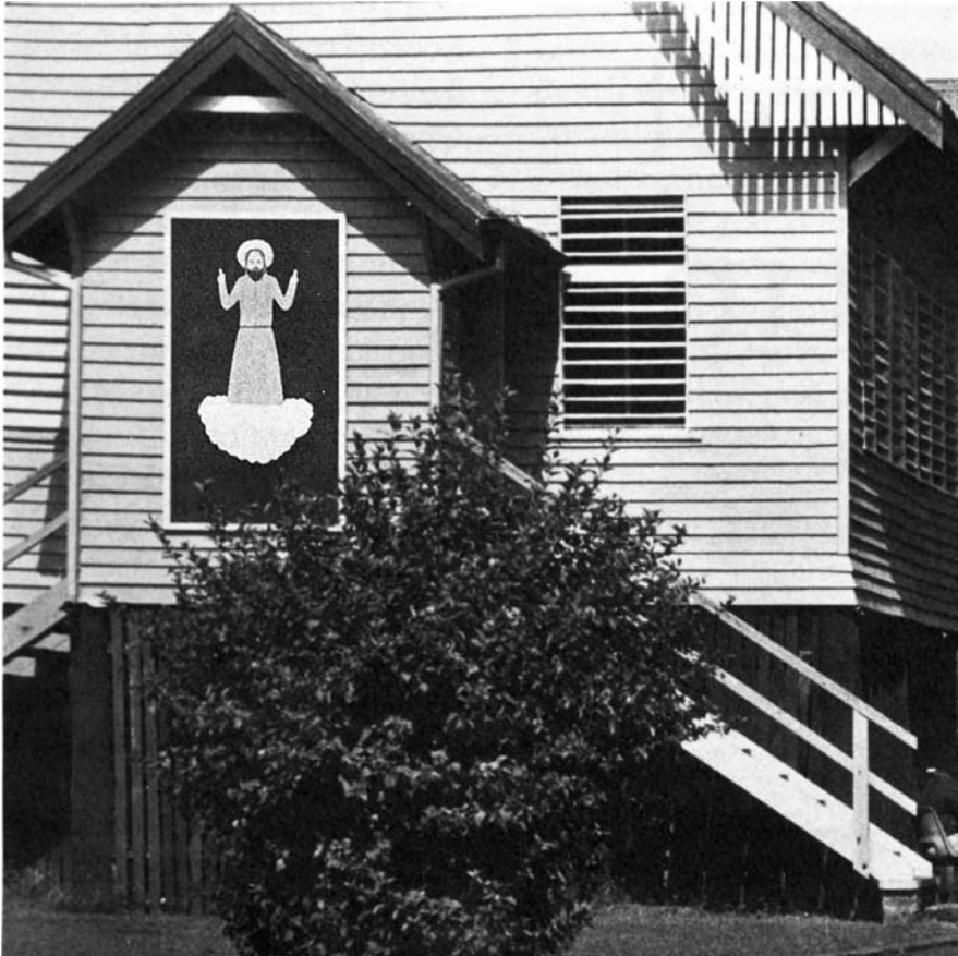
The church. The area underneath was contained between the above ground supporting piles and walled with open palings. This made the learning space dark but still allowed for the use of video. Photo by Henry Strasburger.
