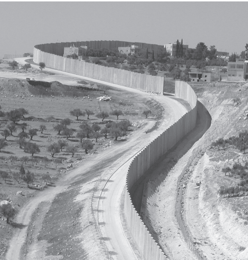
The wall of separation. Israel says it is needed to prevent suicide bombers from crossing over into Israel. Palestinians say the barrier is separating farmers from their land and children from their school. Photo: EAPPI/Jeremy Routledge
