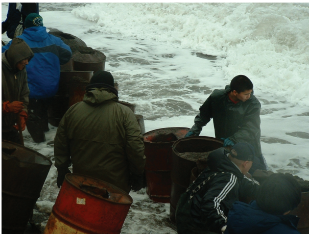
Photo 1. Kivalina residents build an emergency sea wall. Photo courtesy of Millie Hawley
