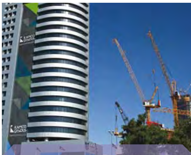
Kuwait City: skyscraper under construction.
