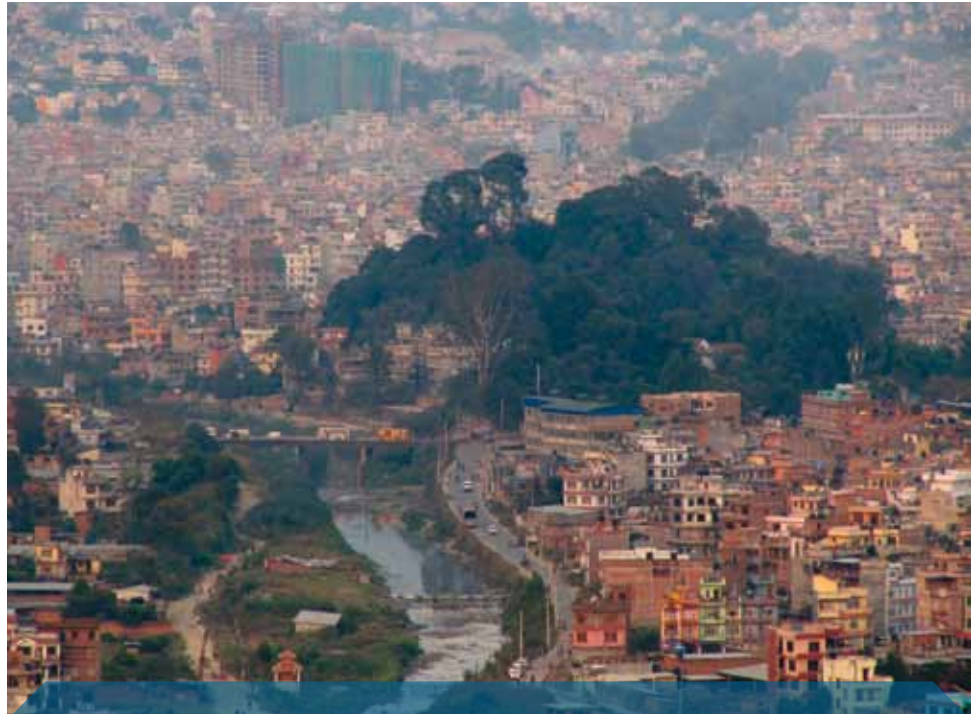
Kathmandu, Nepal: the relentless urban sprawl of the Kathmandu Valley. The Vishnumati River is surrounded by suburbs which have sprung up in recent years. With few building regulations, the city keeps on growing, as many look for a better life in the city than in the countryside. The result is environmental chaos with severe noise, air and water pollution problems.
