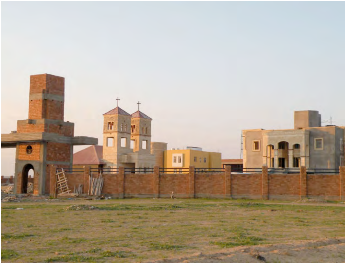
Figure 2. The new Catholic compound under construction in Ankawa, Iraq
