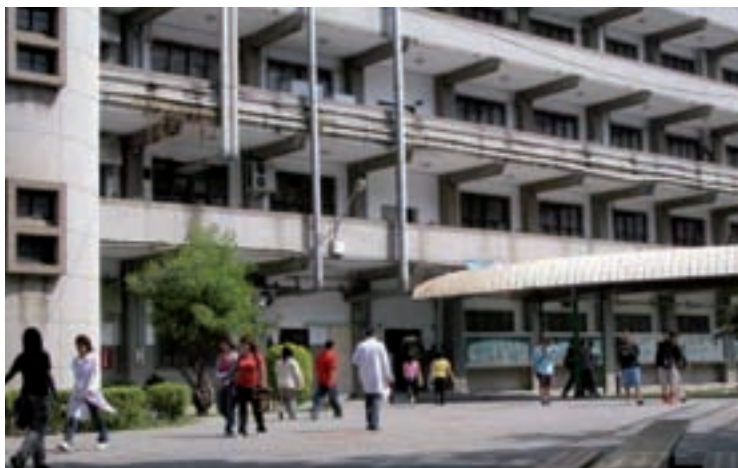
Chung Shan Medical University Hospital enclosure (Taiwan)
