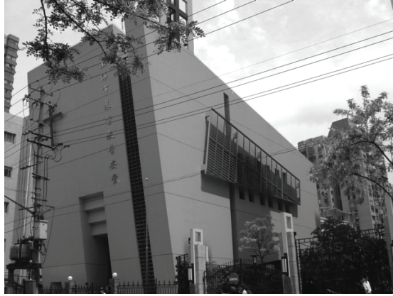
Fig. 5. The Exterior of Pu An Church.
