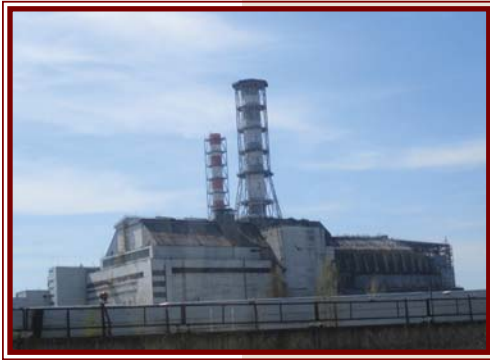
Photo of reactor #4 of the Chernobyl Nuclear Power Plant taken on April 25, 2012. (Source: USC)
