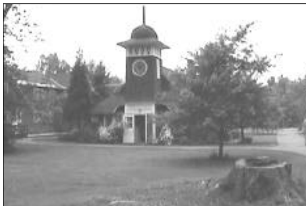
Goddard Clock House building.
